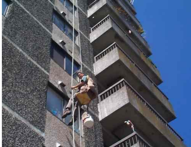
Wall and Window Review using a boatswain's chair
