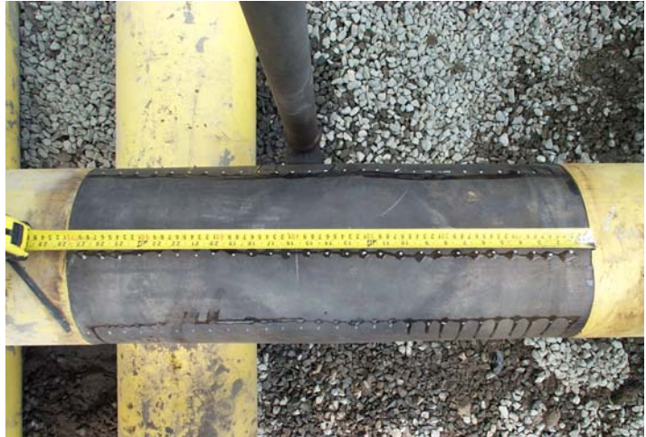
Ultrasonic thickness inspection grid on steel pipeline
