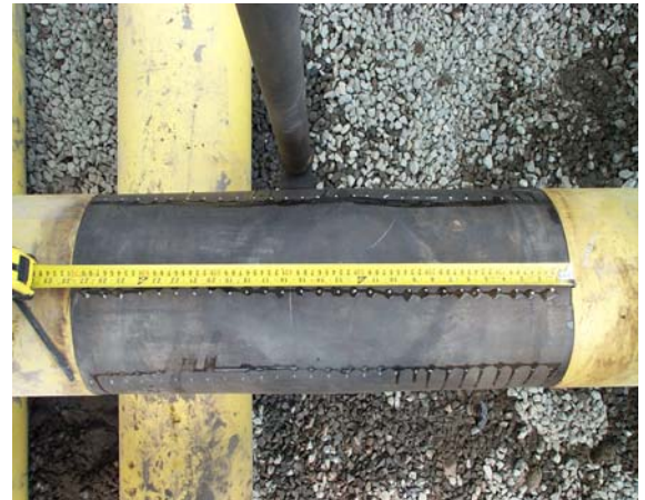
Ultrasonic thickness inspection grid on steel pipeline
