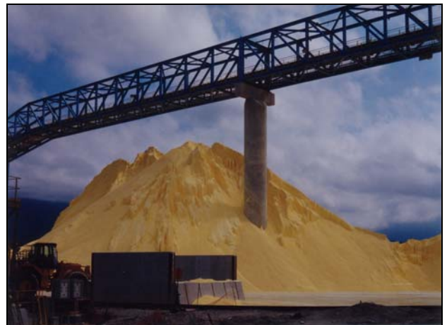
Vancouver Wharves - Berth 4/5
