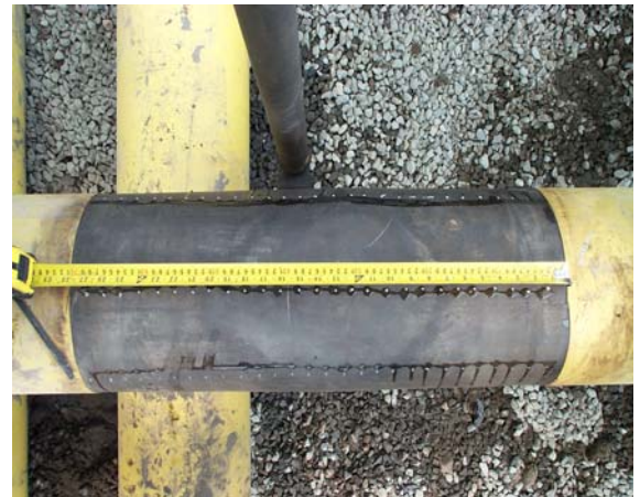
Ultrasonic thickness inspection grid on steel pipeline
